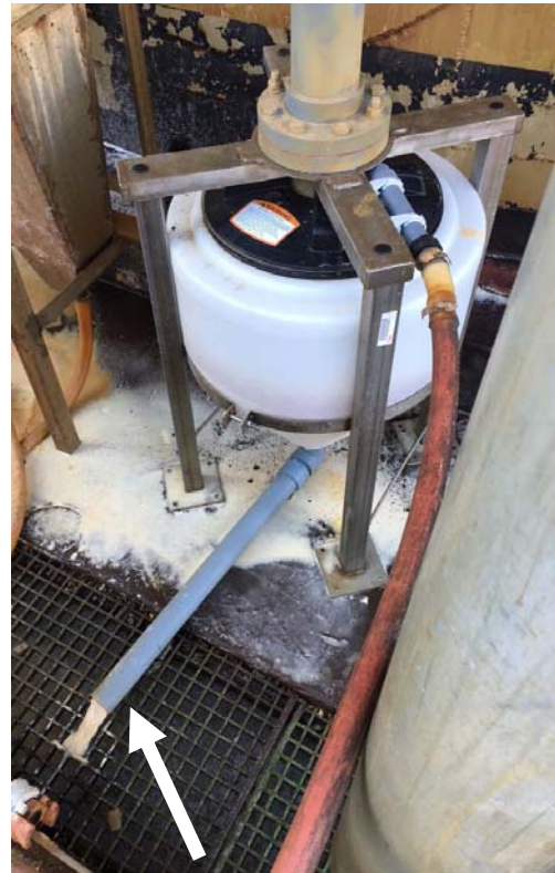
Gravity drain to trench/sump
